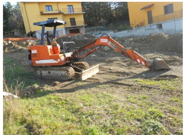
Figure 7. Mini Excavator situated on 21 and 24 November 2014
